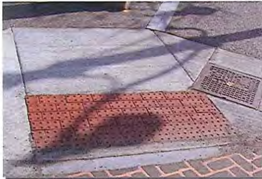
Detectable Warning Field at Curb Ramp Rochester, NY
