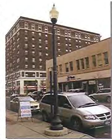
Existing Pedestrian Light Post City of Jamestown
