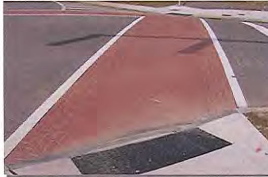
Colored and Textured Crosswalk with Reduced Vibration Zone Buffalo, NY
