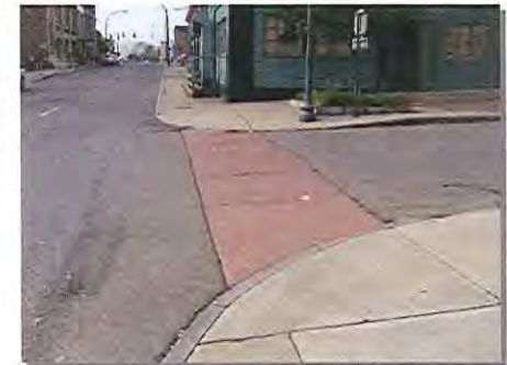
Existing Colored Crosswalk Cherry Street, Jamestown, NY
