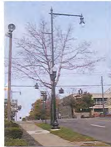
Existing Dual-Purpose Light Post City of Jamestown
