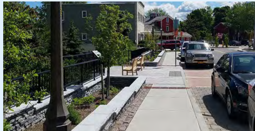
This project in Williamsville, NY, demonstrates multiple green infrastructure strategies, including permeable pavers for the parking lane and bioretention planters as part of the streetscape that capture stormwater and reduce runoff. Strategies like this also help create a more attractive environment.
