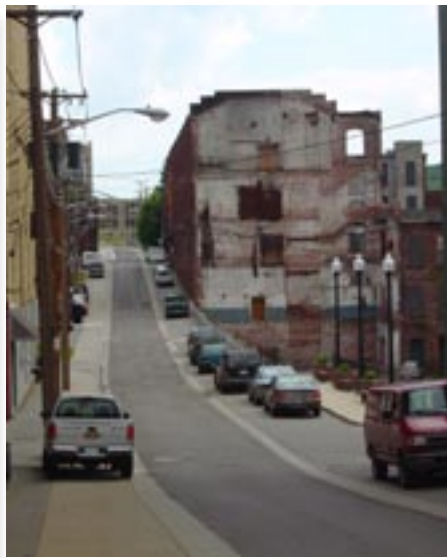
Existing conditions on First Street.
