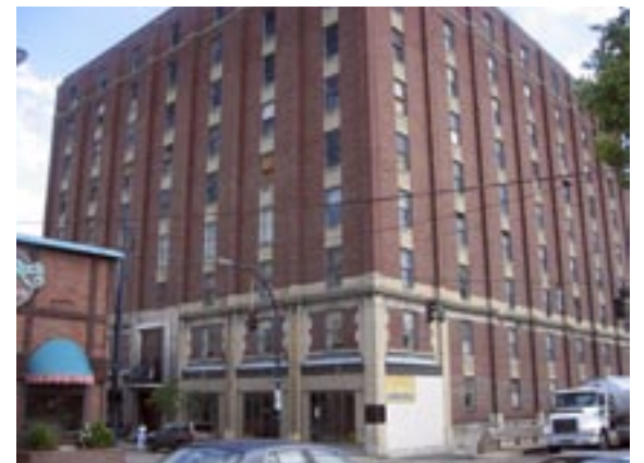
Reusing the Furniture Mart building will play a key role in bringing new life to the West End.
