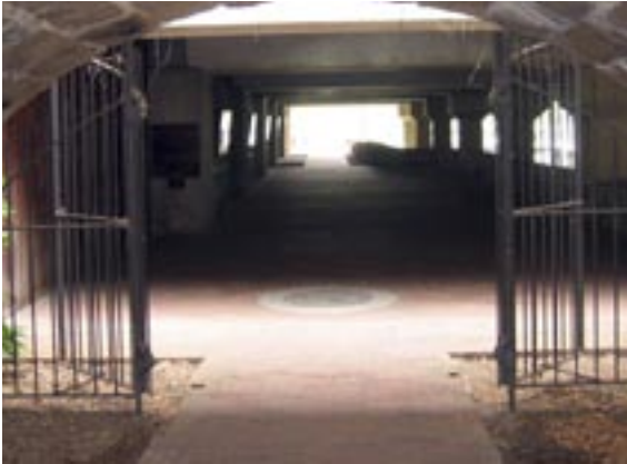
Richmond, Virginia, has created pedestrian walkways that link to the waterfront below rail lines and roadways.
